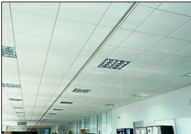
Single and double slot CD diffuser at the DSS office, Newcastle
