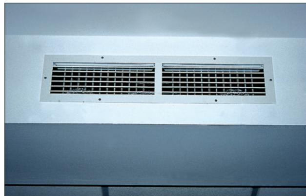
*All models are available with opposed blade volume control dampers operable from the face of the grille and can also be supplied with a wide selection of plenum boxes.*
